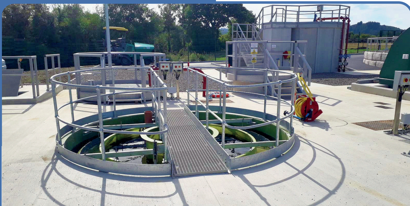
Two number 4 metre diameter FST tanks on a site in Ireland.
