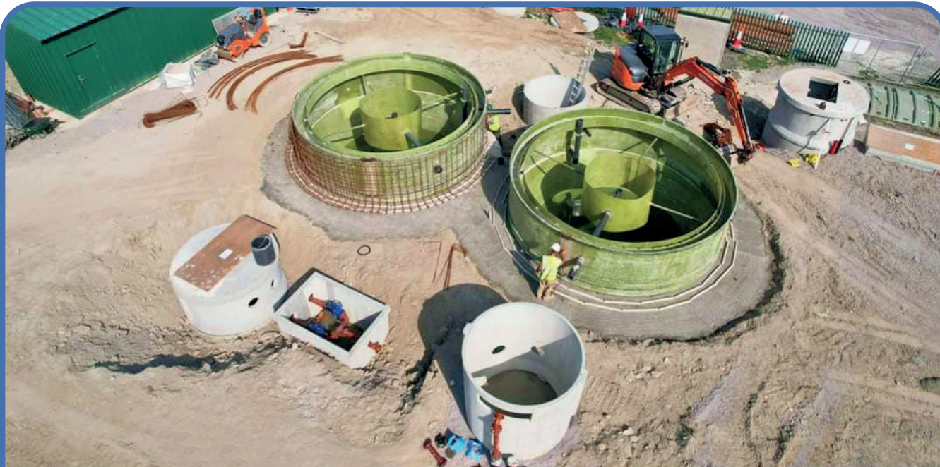
Two number 6 metre tanks being installed.
