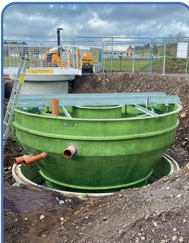
4 metre diameter tank under construction on site.
