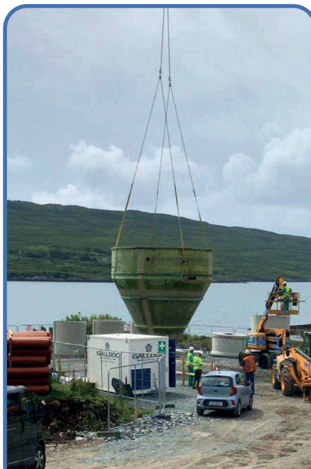
6 metre diameter tank being lifted on site, ready for placing into excavation.
