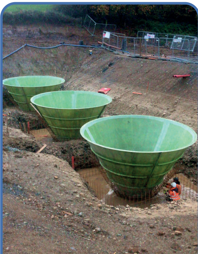
Three number cones installed ready to receive the top sections.
